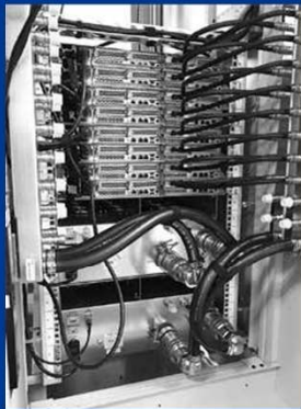
Direct Liquid Cooling System
